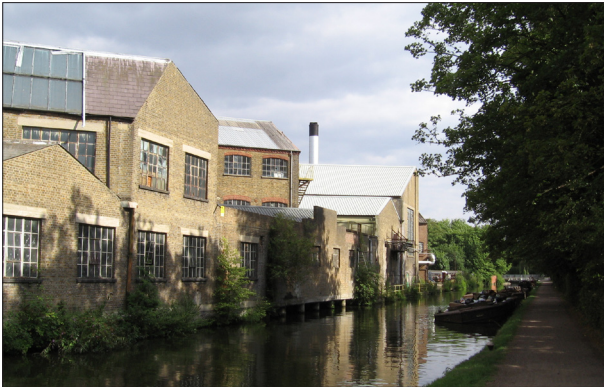
Former SAPPI Mill - Hemel Hempstead
